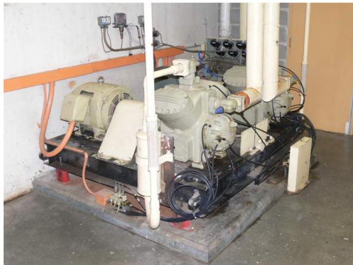
Figure 3. Open Drive R22 Compressors
