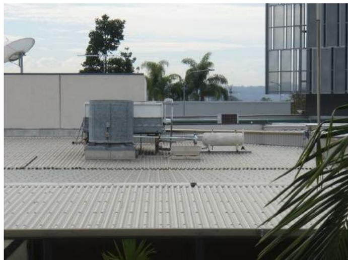
Figure 5. Remote Air Cooled Roof Mounted R22 Condenser
