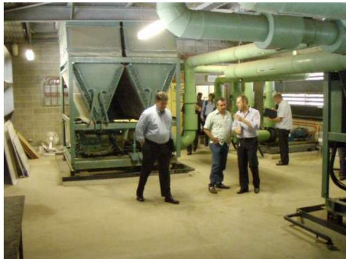
Figure 1. Existing Roof Top Plant Room with Two Air Cooled Water Chillers and Chilled Water Pumps
